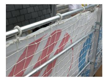
The floors, handrails and netting are installed on the consoles and guardrails to make sure that the scaffolding is safe to work on.
